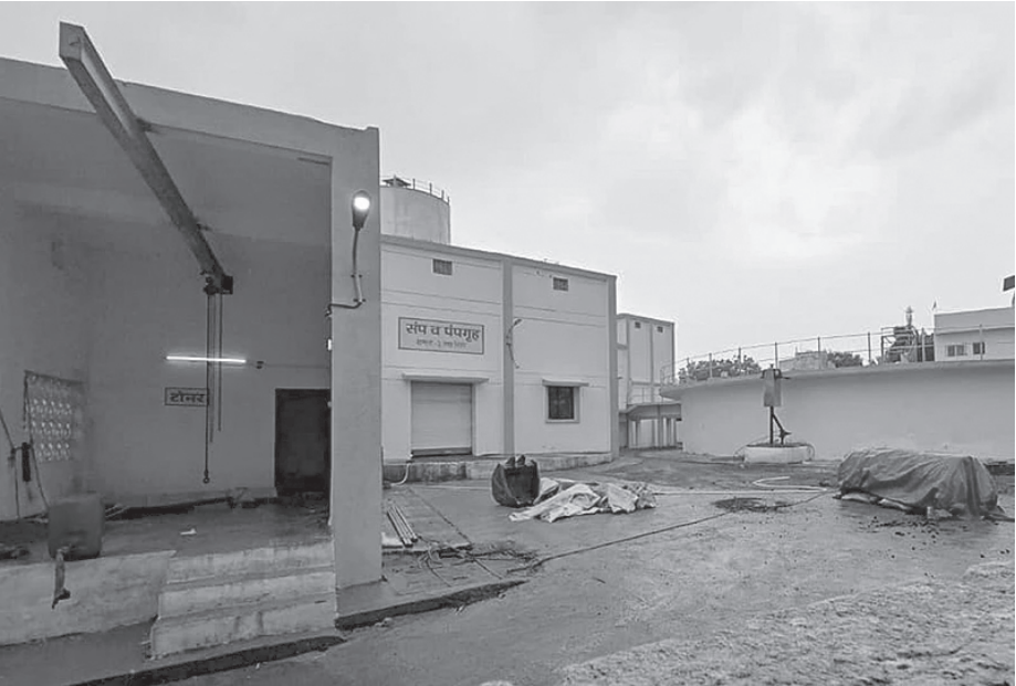
Premises of a water treatment plant following a chlorine gas leak, at Godhani village, in Nagpur.
